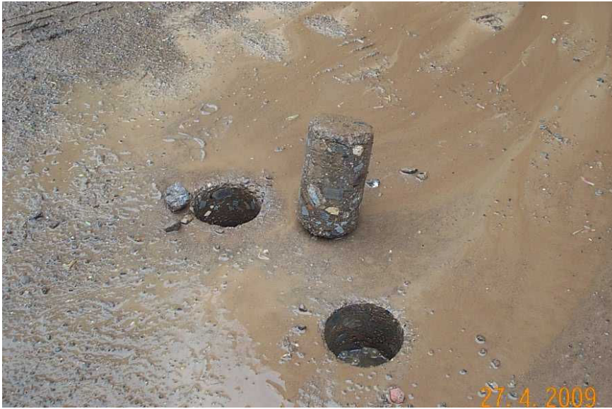
Figure 7. Core of stabilised soil material
