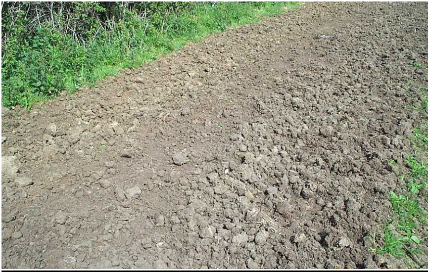
Figure 12. Close-up of surface of stabilised cow track
