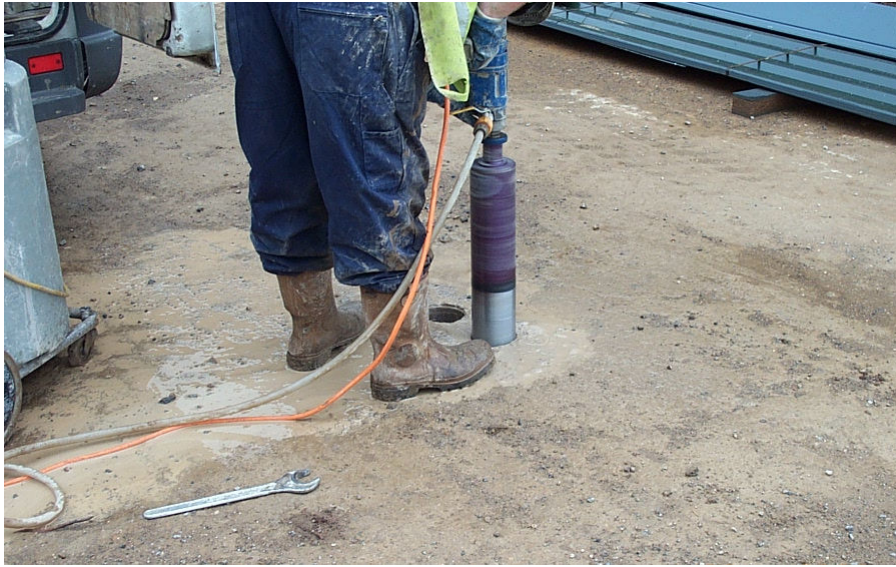
Figure 9. Cores taken from an area of yard containing a higher percentage of aggregate – Warren Farm
