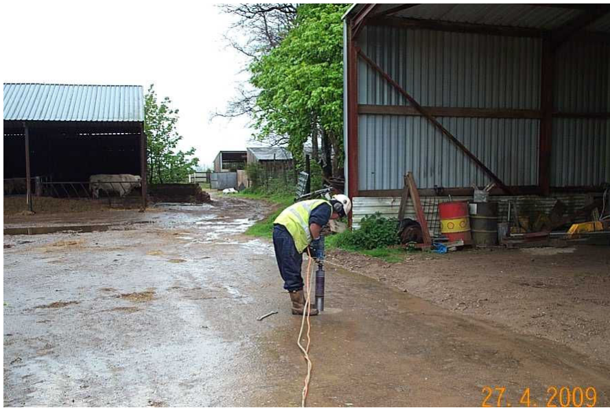
Figure 5. Coring at Warren Farm yard area
