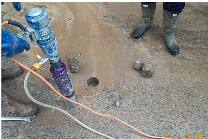
Figure 6. Coring equipment showing core removed
